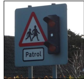
Wig-wag lights can be mounted below the sign assembly or at the side usually as part of a backing board.
